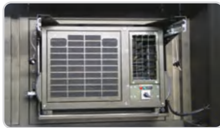
High performance air conditioning unit is used for heating and cooling of the living area. The air conditioner has a maximum cooling capacity of 4.9 kW which is performed as a combination of sensible and latent cooling. The air conditioner can adopt to ambient temperatures from -32° to +60°C.
